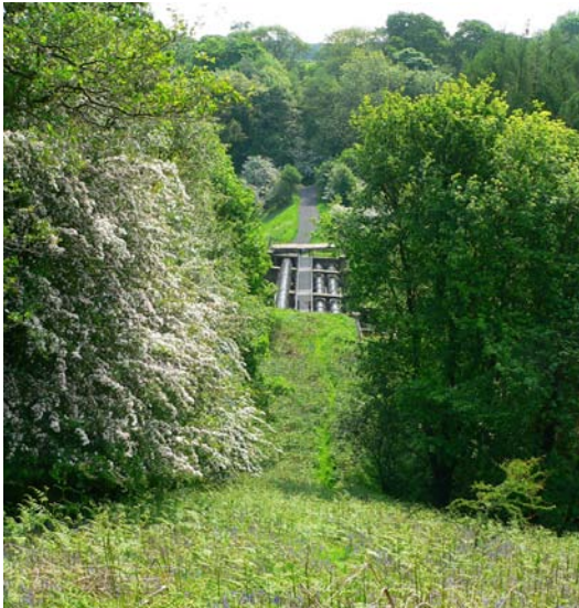
The Brock Siphon
